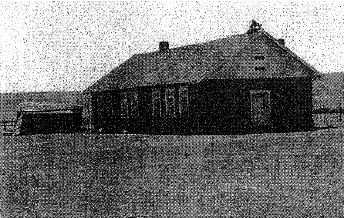
Figure 53: COLONIA GARCIA. Abandoned Mormon School house. Consists of one room.
