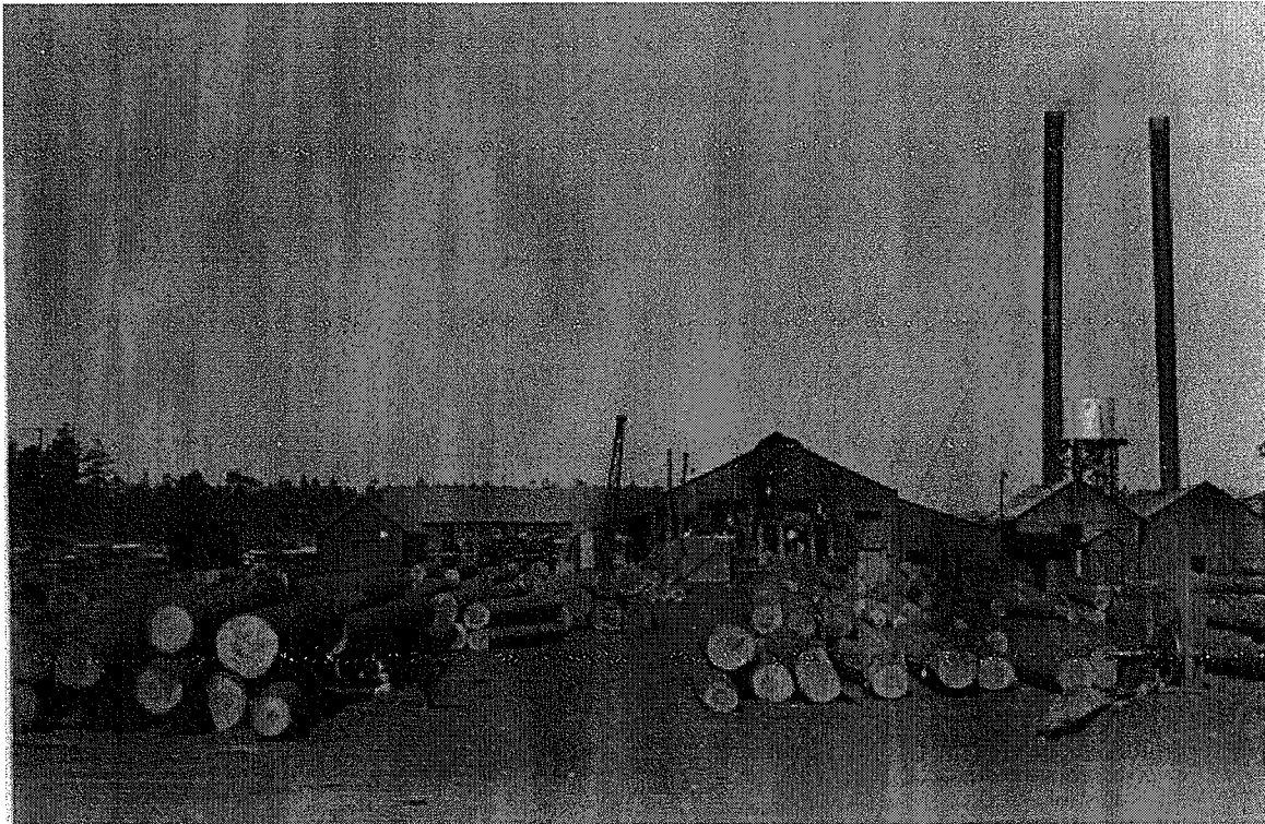
Figure 34: LUMBERING IN THE SIERRA MADRE MOUNTAINS. The saw mill at Largo. The logs are pulled into the saw shed by chain and skids.
