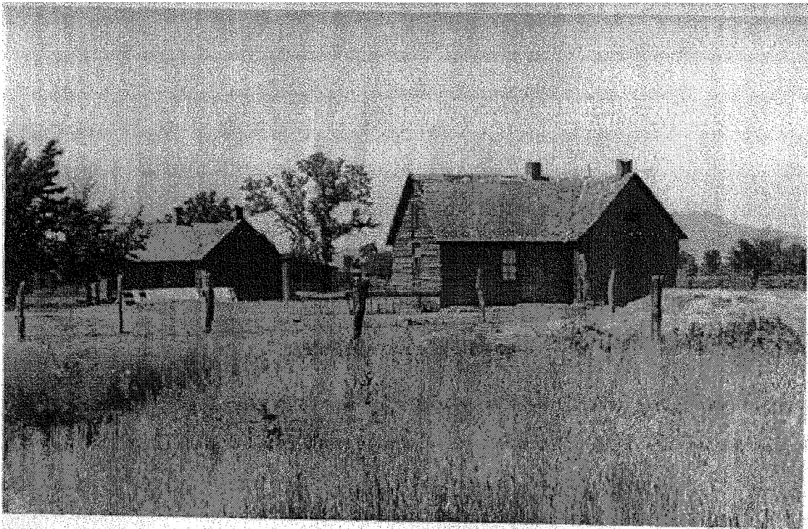
Figure 24: HOUSES IN COLONIA DUBLAN. Wood and adobe home built by one of the first Mormons to settle in Colonia Dublán. Now Inhabited by Mexicans.
