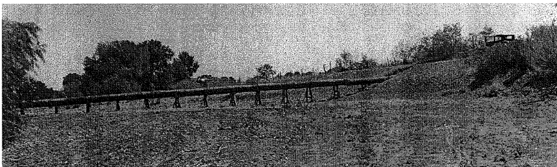
Figure 74: IRRIGATION WATER. This flume is built across the Río Casas Grandes during the spring to bring irrigation water from the lakes to the San Jose tract. It is made from oil drums. When the rainy season begins and water begins to come down the river the flume is dismantled.
