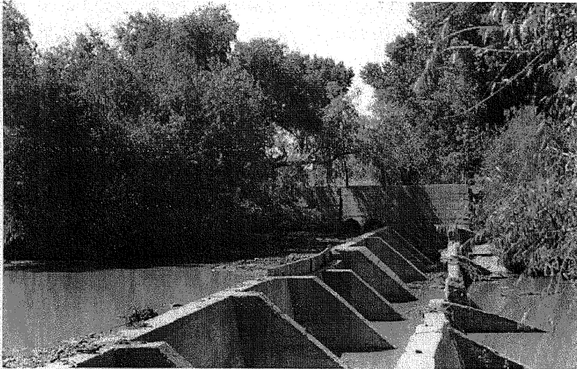
Figure 75: IRRIGATION WATER. A dam to divert the river water into the pipes in the center of the picture. The water flows to the San Jose tract, which is just across the river from Dublán.
